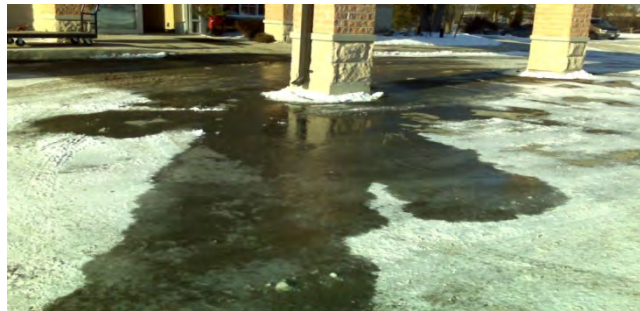
Figure 42. Improperly designed drainage from entrance to nursing home. (Photograph by Bob Hodgins)
