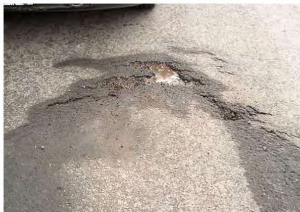
Figure 45. Poor condition of pavement promotes loss of chloride by infiltration to the subsurface. (Photograph by Bob Hodgins)
