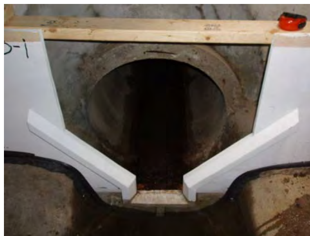
Figure 38. Compound Weir Installed
